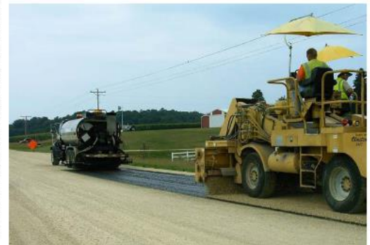
Otta Seal Const. 2007, Olmsted County CR58
